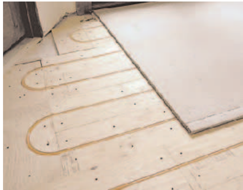
Figure 7. For tiled areas, cement backerboard is installed on top of the Climate Panels.
