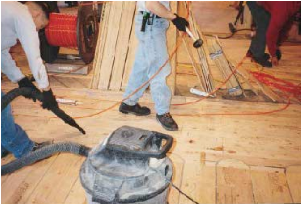
Figure 3. Panel grooves must be carefully vacuumed to remove any debris that could cause the tubing to protrude.
