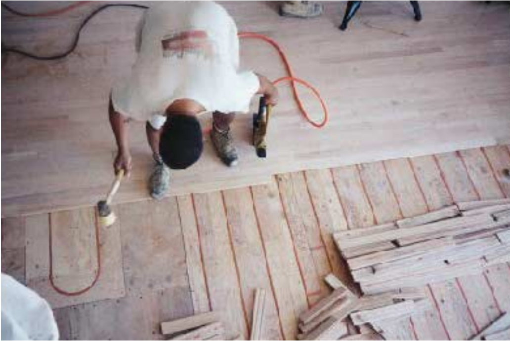
Figure 6. Hardwood strip flooring can be nailed directly to the Climate Panel. Leaving out the customary felt paper makes it easy to avoid the tubing when nailing.
